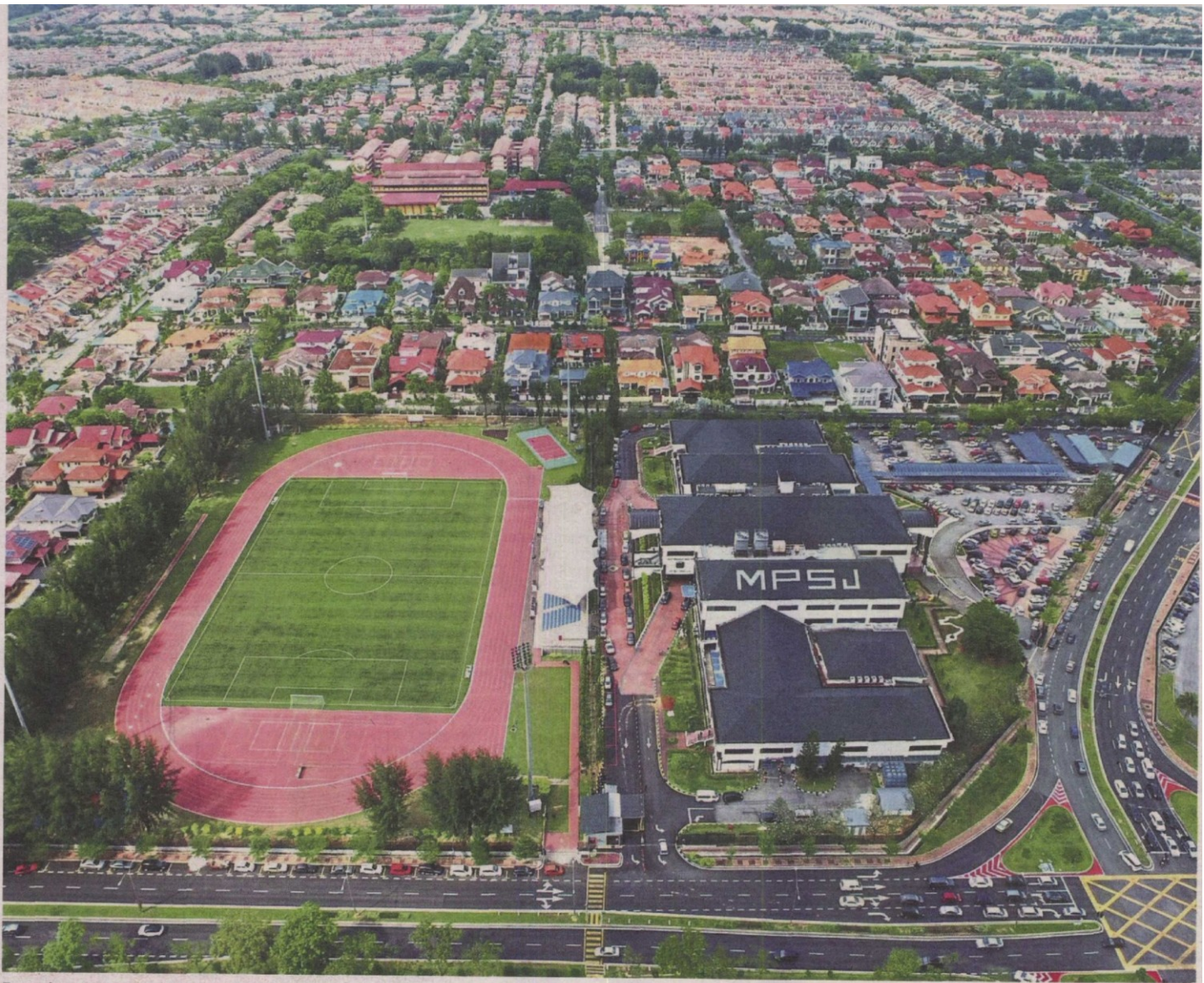
Exemplary progress: A bird's eye view of the MPSJ building and its surrounding neighbourhood. — IZZRAFIQ ALIAS / The Star
